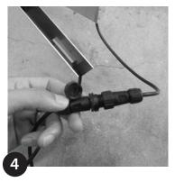
Make connection and feed cables into ground box ensuring that it won't come under strain or hinder product installation.
