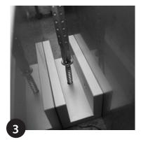
Using the appropriate screws for the mounting material, screw the ground box into the recessed slot via the mounting brackets pre-installed into the ground box.
