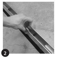
Insert ground box into recessed slot. If self-tapping screws cannot be used, use the ground box to mark the screw locations to pre drill holes.
